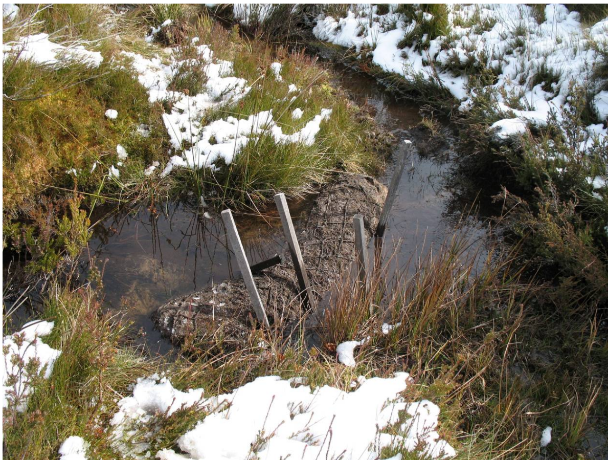
Figure 7-4 Restoration works at Ginini Flats Wetland Complex showing a coir log used to dam a small stream
