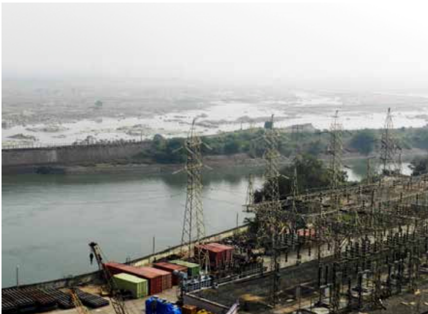
Burla Power Station
