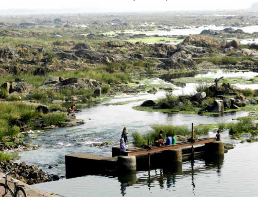
View of Dam Dyke
