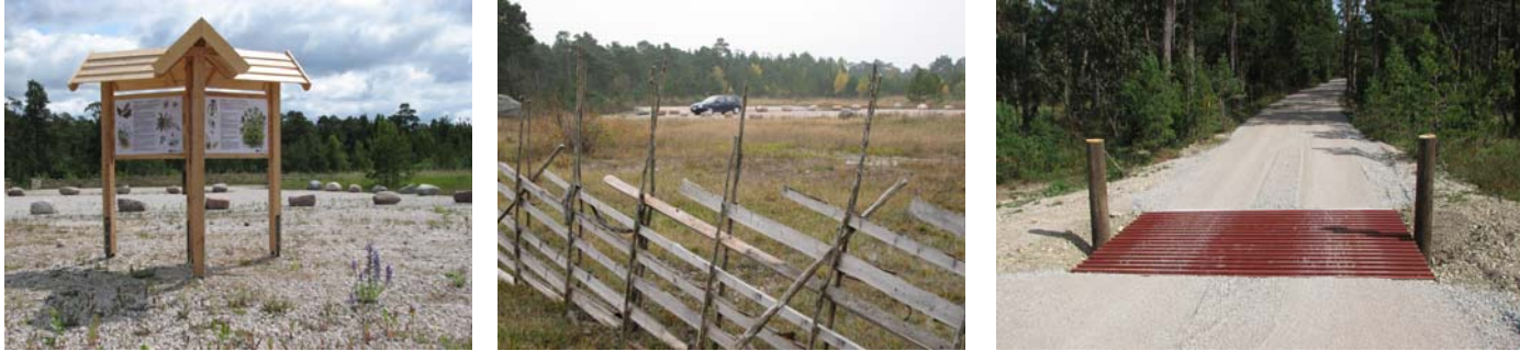
Pictures of constructions made in the LIFE-project at the information place; Information boards, Parking lot with a traditional Gotlandic fence, and a cattle grid.
