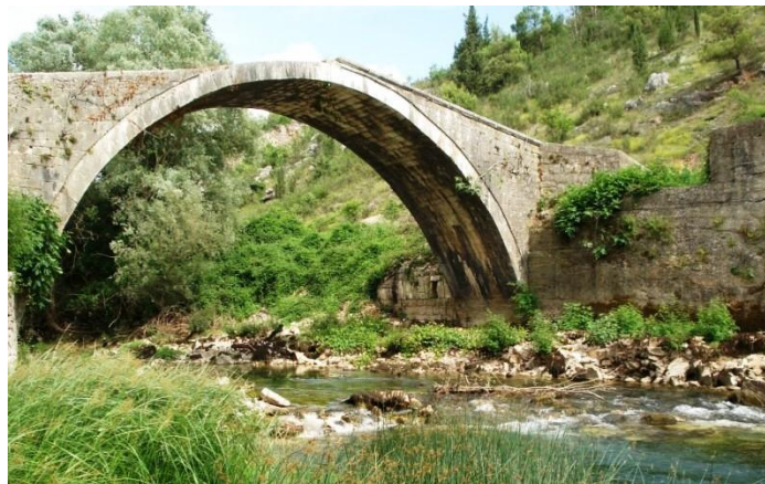
Figure 2.29: Bridge in Klepci
