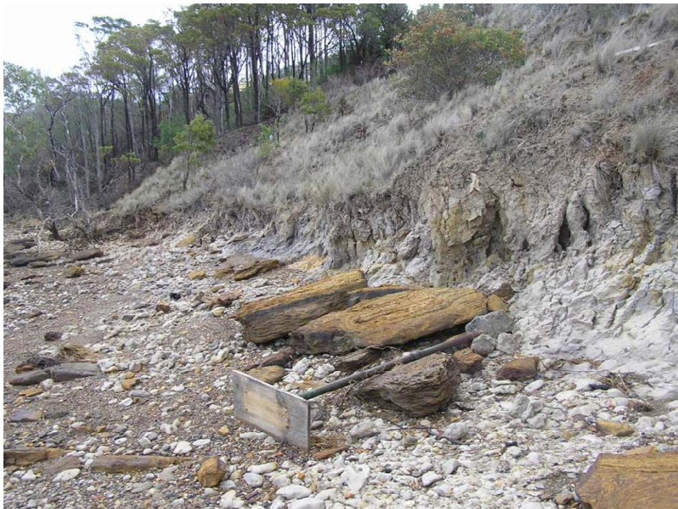
(b) Erosion at Shark Point Road, Penna (H Dunn May 2009)
