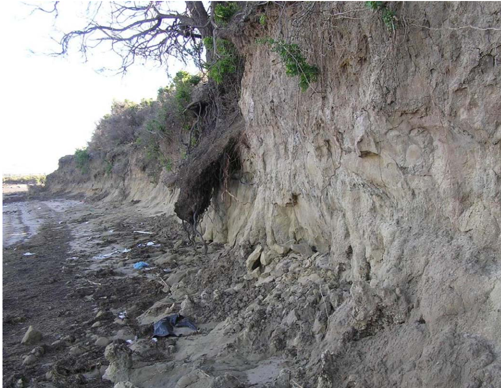
(a) Erosion at Sorell Point (H Dunn May 2009)
