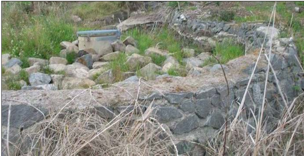
Figure 7 Solid waste trap beside Orielton Lagoon at Midway Point
