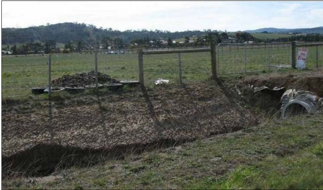
Figure 6 An eroded open drain in Sorell discharges directly into Orielton Lagoon
