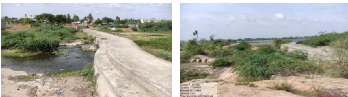
Weirs of Nanjarayan Tank
