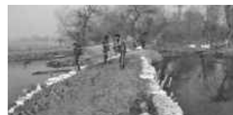
Plugging of breaches and restoration of marginal bunds in Hokersar Wetland
