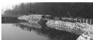
Plugging of breaches and restoration of marginal bunds
