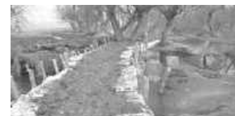
Plugging of breaches and restoration of marginal bunds in Hokersar Wetland
