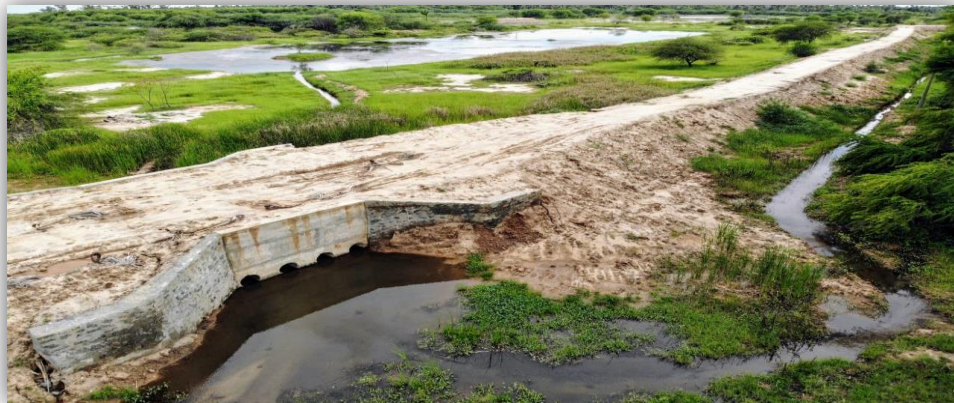
CONSTRUCTION OF HUME PIPE CULVERTS
