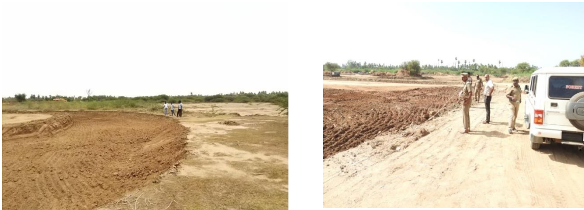
DEEPENING & DESILTING WORKS
