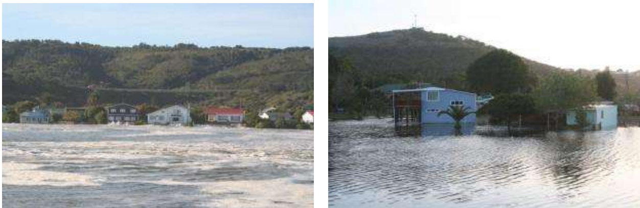
Figure 3.4 Coastal storm overtopping sand berm at mouth and causing flooding at Groot Brak, 1 September 2008 (Source: J Kriel, DWA)
