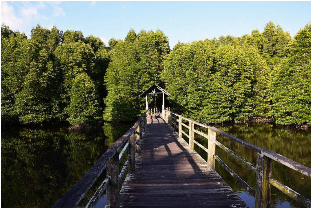
Plate 2-7: The boardwalk extends for 1.5 km into the mangrove
