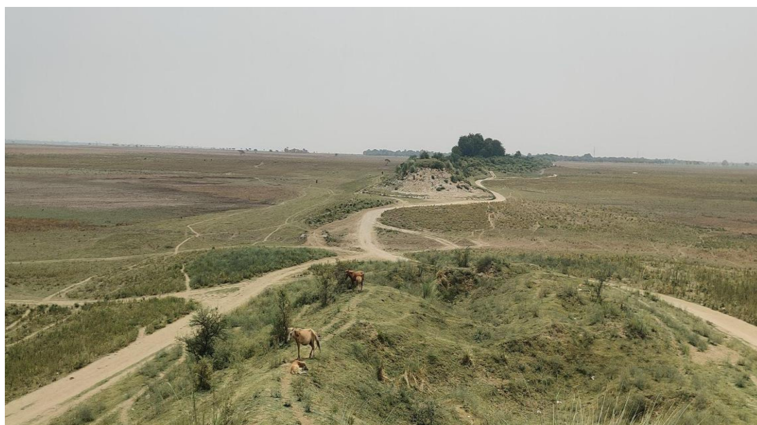
Embankment breach of approx. 250 m at Isharpura village (Flood water enters from River Ganga to Sunki Suhiya-25°41'57.8"N 84°23'37.9"E)
