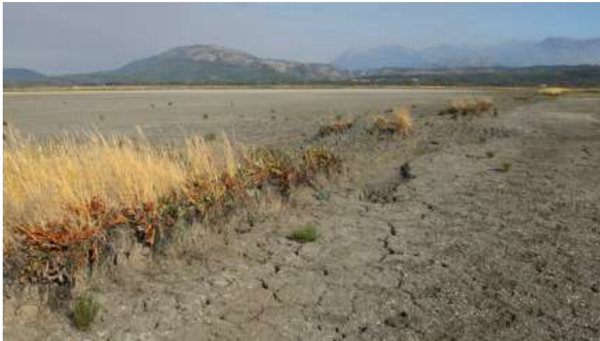
Figure 12.2: Inner dikes in nature protection priority areas can be left to natural degradation, like shown on this picture.
