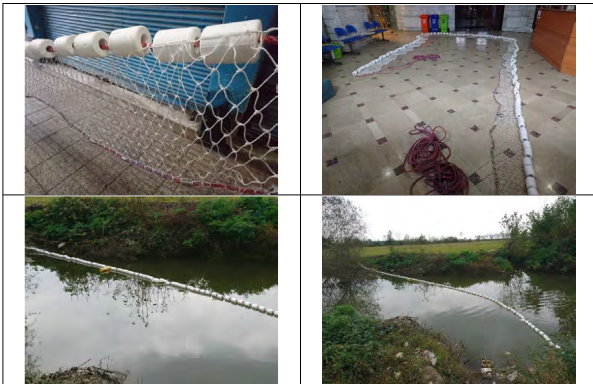
Figure 6.7-11 River Waste Trapping Net Installed in the Wetland
