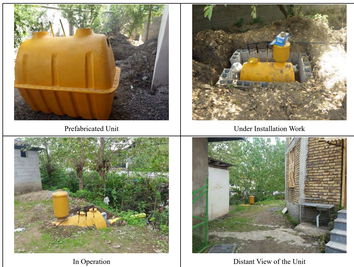
Figure 6.6-8 On-site Sewage Treatment Unit in Mobarak Abad Village
