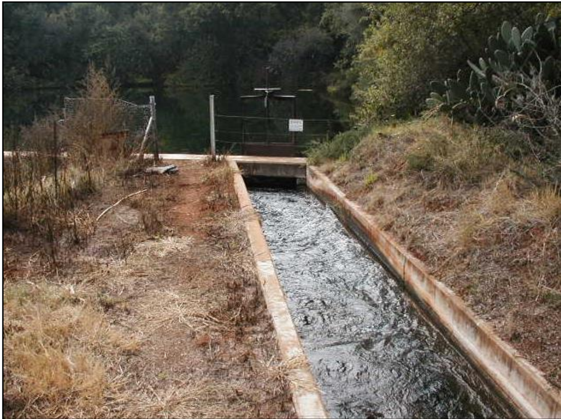
Figure 55: Gerhard Minnebron dolomitic eye and water abstraction canal diverting a substantial proportion of the water for agriculture use
