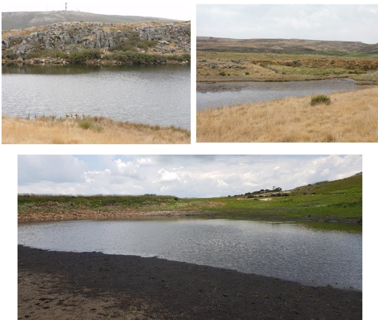
BMU11: Dam 1 (top) and Dam 2 (bottom) on the Farm De Berg.
