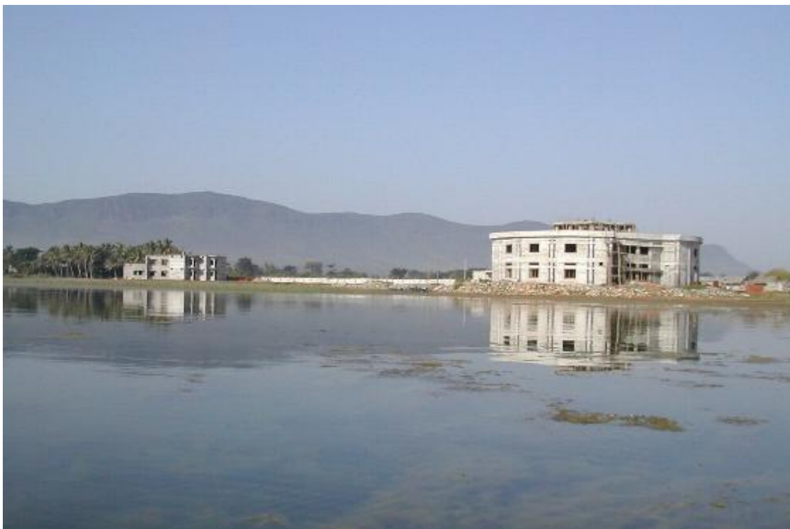
View of wetland education and research centre and residential facility for researchers (under construction)
