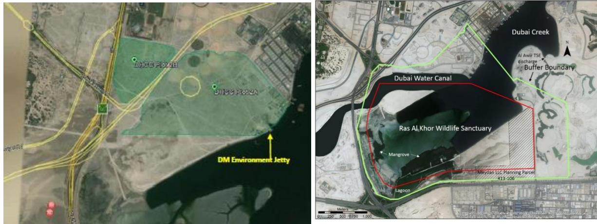
Figure 7. Prior to excavation of Dubai Water Canal (3 March 2000) 35 on right and completed canal on left within boundary of RAKWS and buffer zone.
