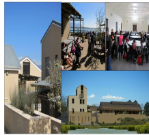
False Bay Nature Reserve Headquarters Complex (left), showing community use of the multi-purpose hall and associated courtyard (top centre and right) and Architect's impression of the now completed Complex (bottom right). ( City of Cape Town, 2014 )
